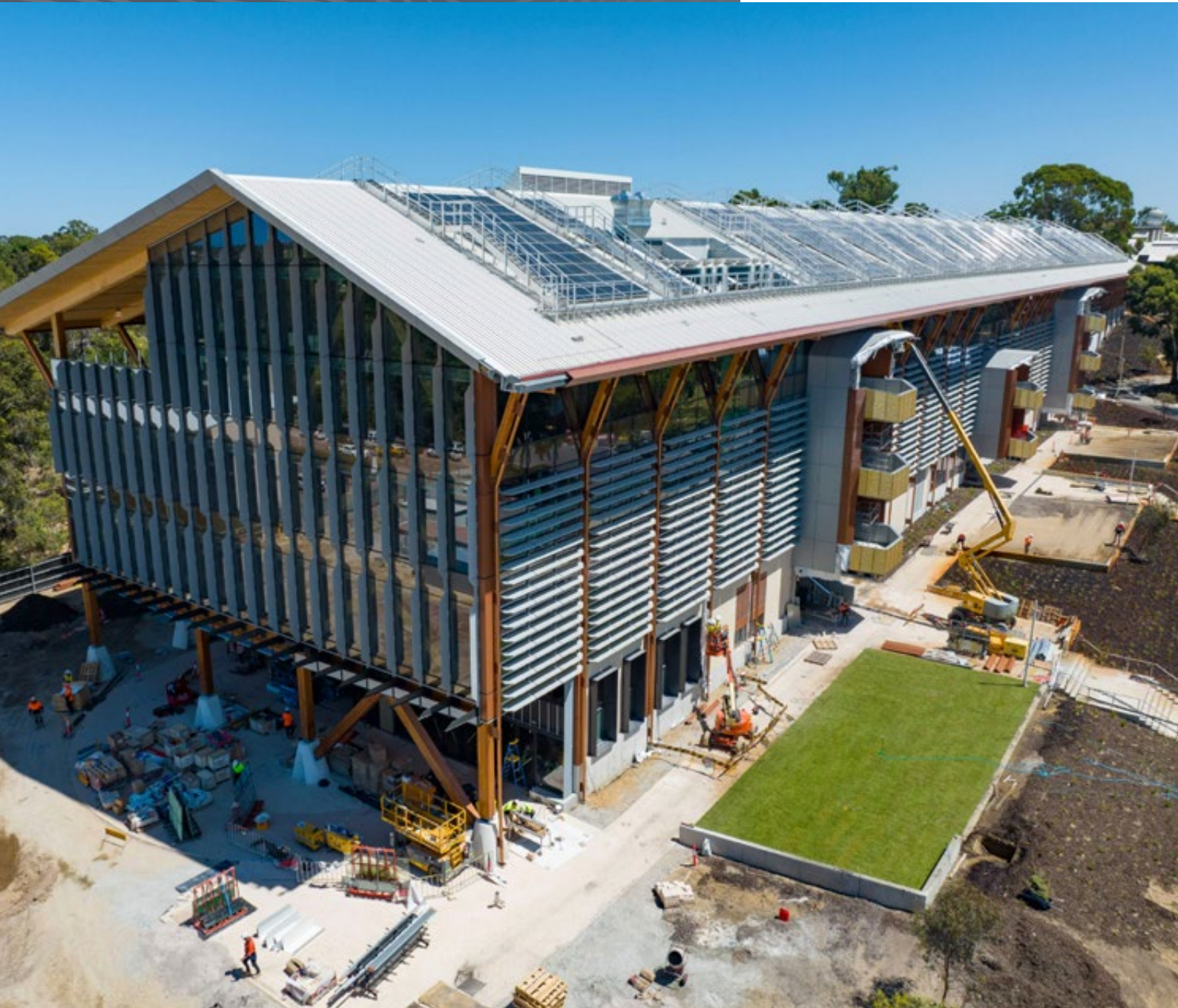
Boola Katitjin under construction in 2022
